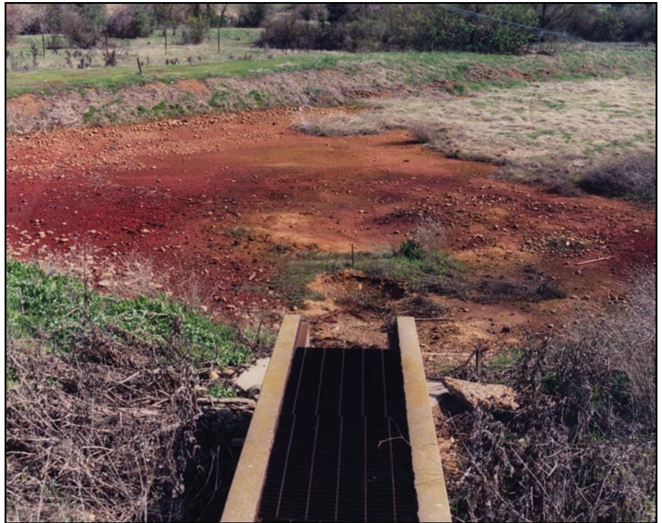
Aerojet-General's 'state of the art' waste treatment plan included this open trench and unlined drainage pond.
