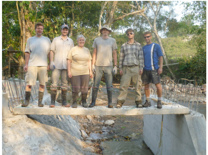
Duane Morris LLP attorney Jeffrey L. Hamera (at left) and Chicagoland Chapter of Engineers Without Borders members Tyler Grau, Nancy Holmes, Dan Atkins, Mark Ward and Joti Baruni demonstrated the load-carrying capacity of a 5-inch, precast deck panel, one part of a bridge EWB built in Canchias, Honduras, last year.
